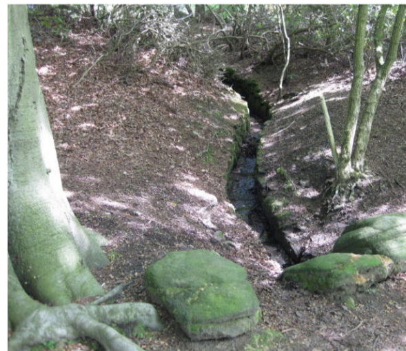
Culvert carrying water from the wheel to Baxter's Pond
